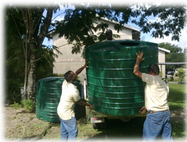
a). Rainwater Harvesting tanks in Schools
