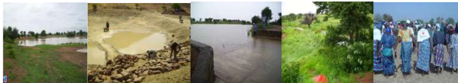
Degraded Reservoir Rehabilitation works Rehabilitated Reservoir Healthy Watershed Happy Community
